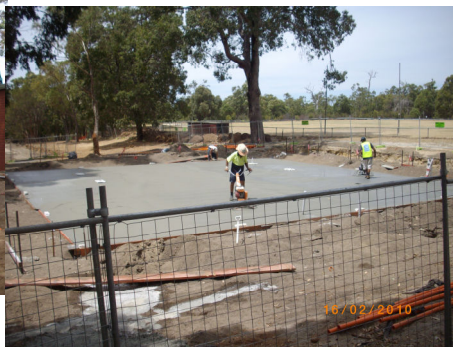
The completed pad this morning
