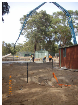
Concrete being applied to the Library.
